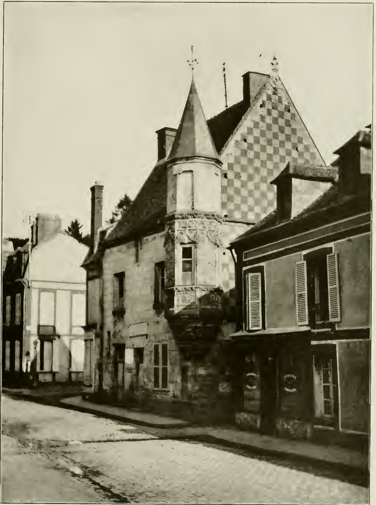
PLATE 59. House at Verneuil, Eure
